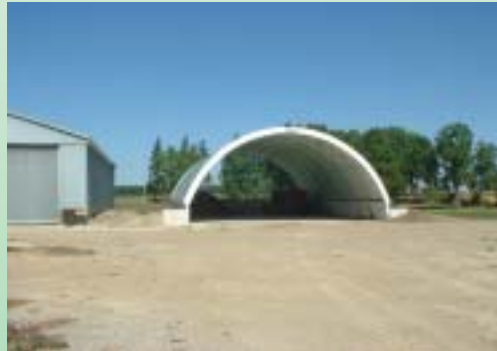
Covered manure storage eliminates runoff from the manure stack, protecting nearby watercourses.
