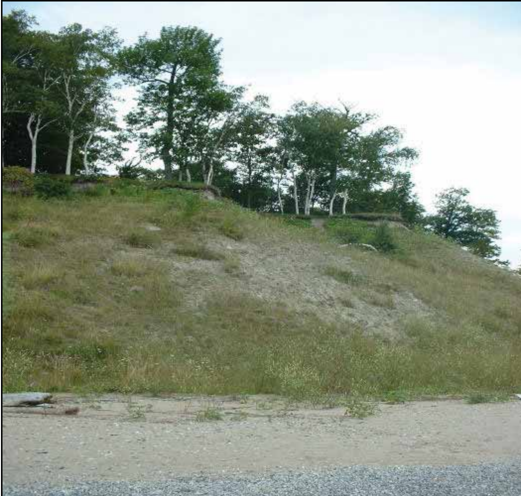
Figure D- An example of a property located within Block 2 where the toe recession was found to be the highest in the study area. Exposed slope, channeling and undercuts at the top of bluff are visible. St. Clair Region Conservation Authority- September 2004
