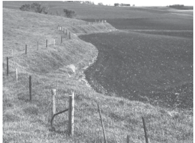
An earthen berm may be an effective method to divert water away from a potential source of contamination.
