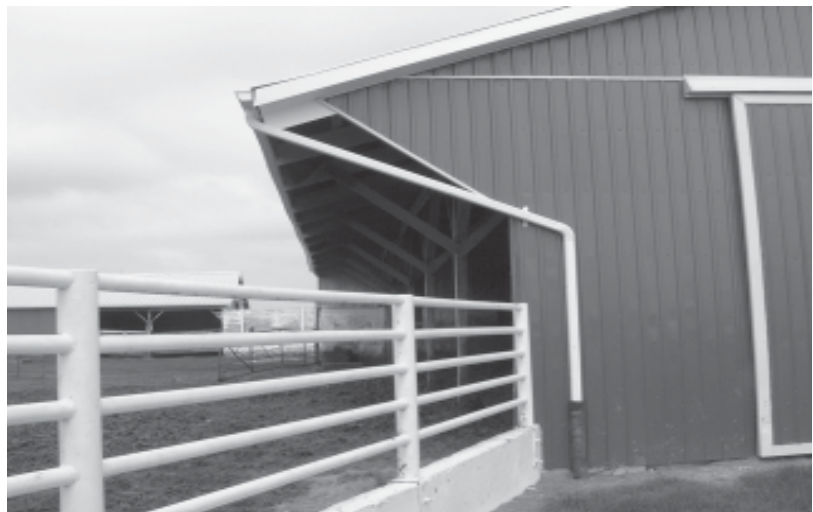
Eaves troughs, diverting water from the roof away from a feedlot, helps to reduce polluted runoff into nearby watercourses.
