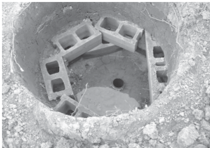
Abandoned wells allows for access of pollutants into the groundwater. These wells should be properly decommissioned by a licenced contractor.
