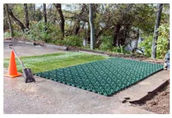
The green parking spaces were constructed by placing a base of course gravel followed by a layer of sand to allow for infiltration. A plastic panel is then installed and back filled with top soil that acts as an anchor for the grass that is planted on top.
