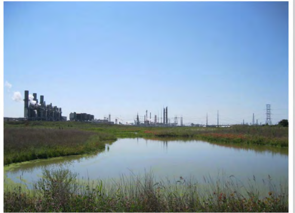
Bowens wetland phase less than a year after construction.
