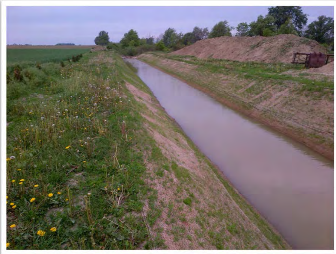
Figure 2. Courtney Drain, Camden drain relocation with more stringent sediment and erosion applied.
