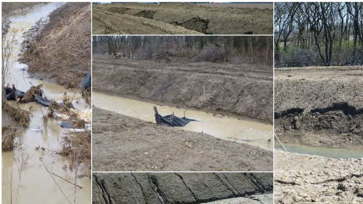
Figure 1. Drain relocation done in winter with in-adequate sediment and erosion control
