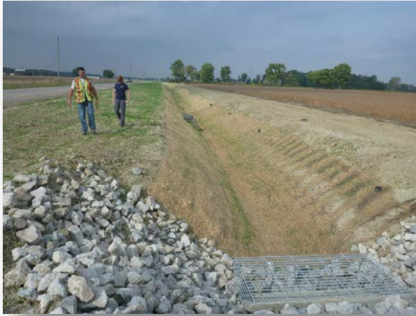
Drain re-location project in Township of Dawn. By using mitigations such as erosion control blanket, seeding of banks and timing construction to allow vegetation to re-establish, erosion is greatly reduced.
