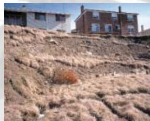
Slope failure
