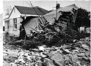
Homes crushed by thousands of gallons of water
