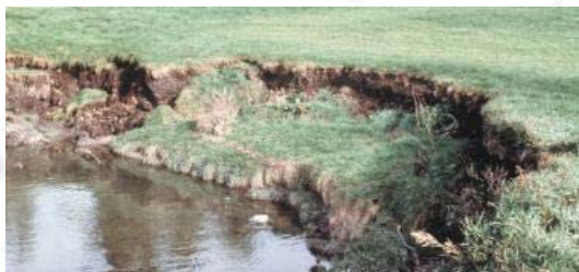
River bank erosion
