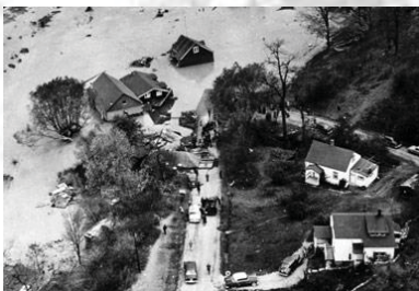
Raymore Drive- houses had to be torn down
