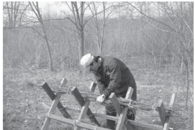
*A fascine is a bundle of live cuttings that is placed into a trench along the streambank and grows to provide vegetative cover and stability to the slope. Cuttings are taken during the dormant season from shrubs of dogwood and willow.*
