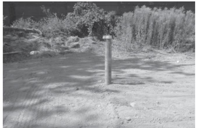
*After - Repaired well with an extended casing 16" above finished level with a proper well head cap.*
