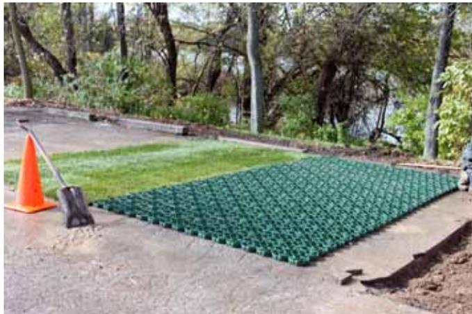
The green parking spaces were constructed by placing a base of coarse gravel followed by a layer of sand to allow for infiltration. A plastic panel is then installed and back filled with top soil that acts as an anchor for the grass that is planted on top.
