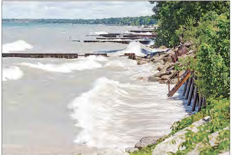
THIS STRETCH OF Bright's Grove shoreline, looking east from the foot of Kenwick Street, is in danger of collapsing in a major storm, engineers warn. As Lake Huron water levels increase so does the need for expensive shoreline protection.
