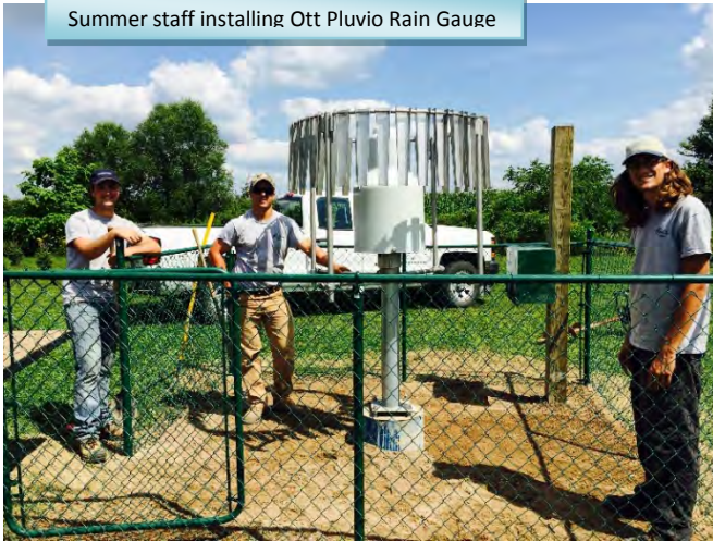
Summer staff installing Ott Pluvio Rain Gauge
