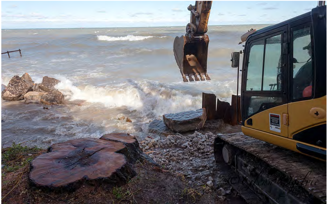
Heavy equipment and crews from Van Bree Drainage & Bulldozing work to shore up the breach with rock and stone. Glenn Ogilvie
