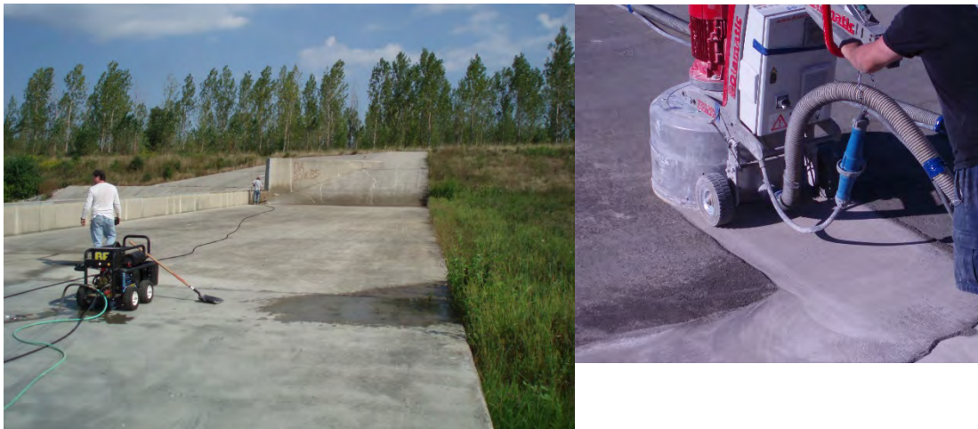
McKeough Dam Outlet crack repair
