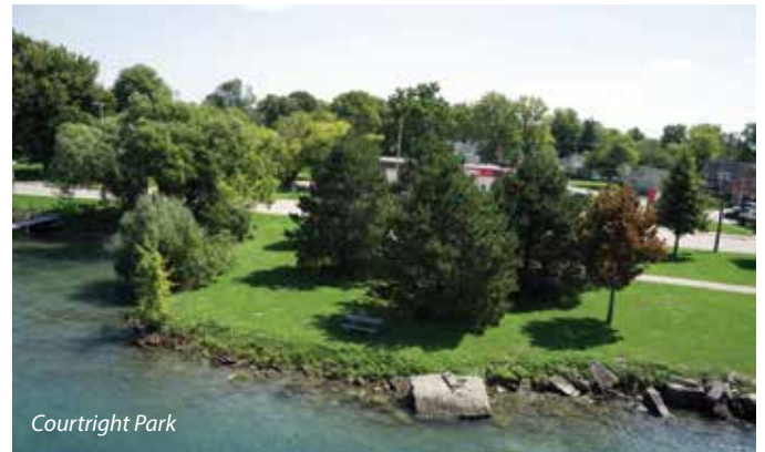
The proposed design at Courtright Park will include an armour stone/rip rap revetment with aquatic planting and gravel beds incorporated along parts of the shoreline.
