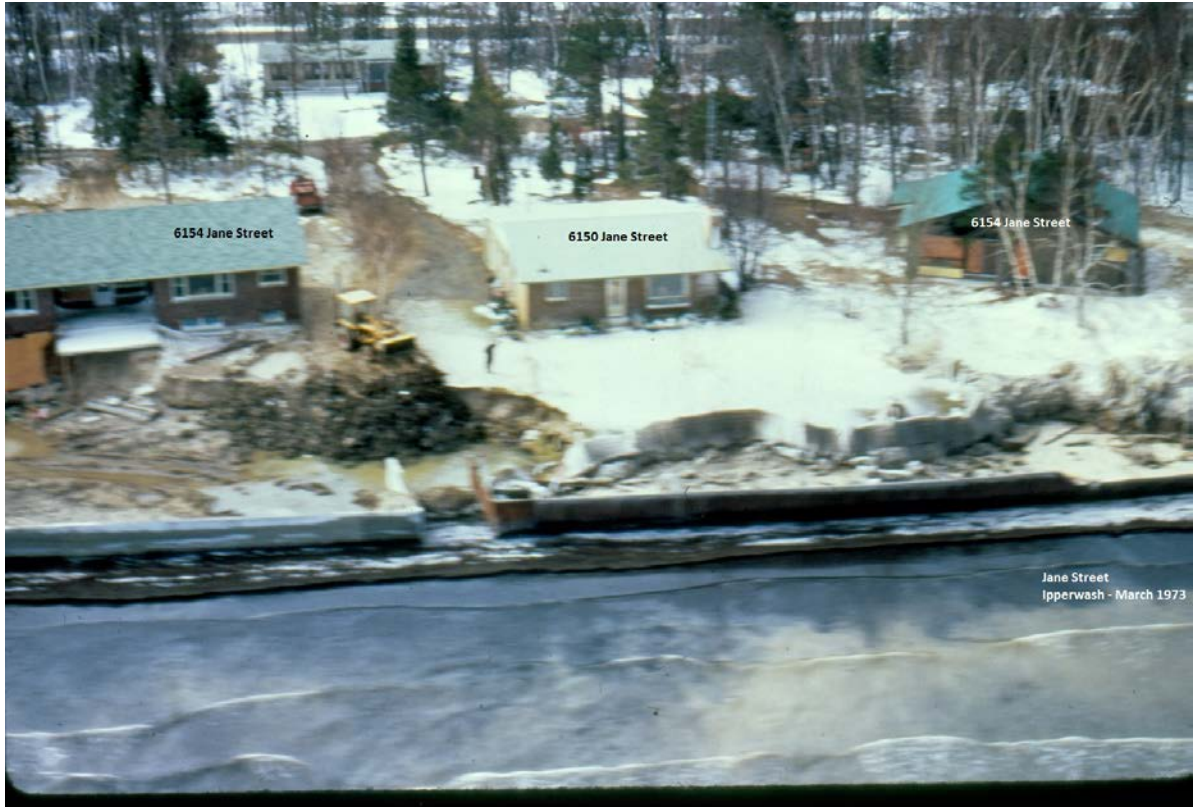
Figure 6.1a March 1973 Scour behind Seawall from Overtopping after Storm Event
