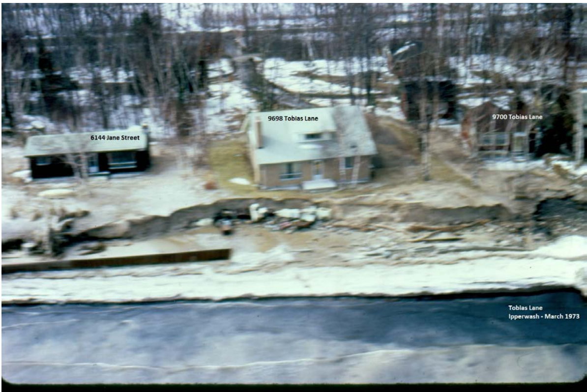
Figure 6.2b March 1973 Scour behind Seawall from Overtopping after Storm Event
