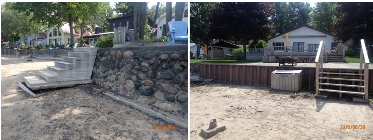
Figure 6.1 Examples of Stone and Concrete Seawall and Steel Sheet Pile Seawall in the Study Area
