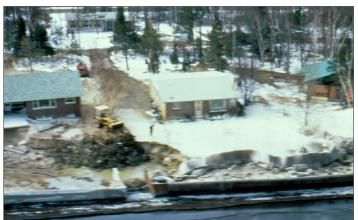
*Seawall Failure: scour behind seawall from wave overtopping after storm event (Jane Street, March 1973)*
