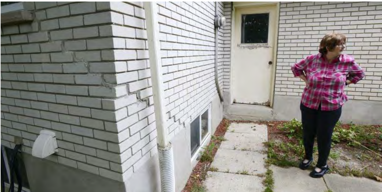
Donna Dobroski's distress: The corner of her house has settled, causing an ugly crack in the brick wall due to erosion into the Red Hill Valley behind her home.
