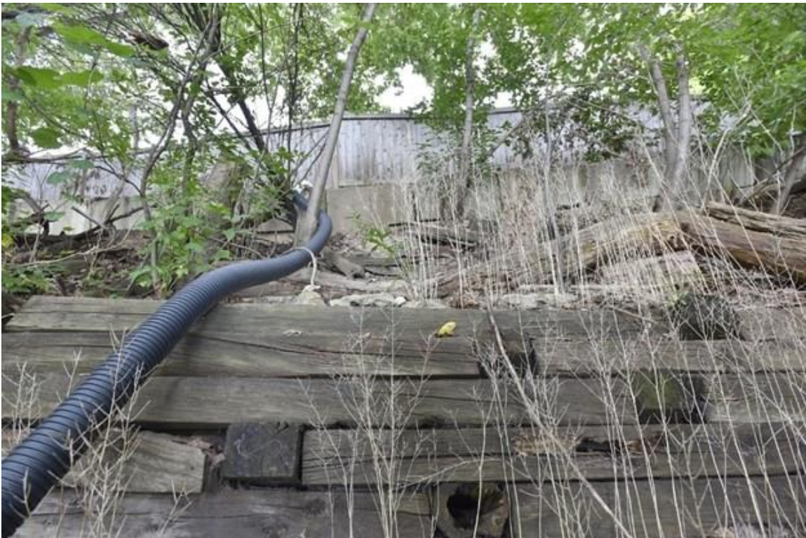
A retaining wall of railway ties was installed behind her Donna Dobroski's house. It was later reinforced with concrete blocks, above.
