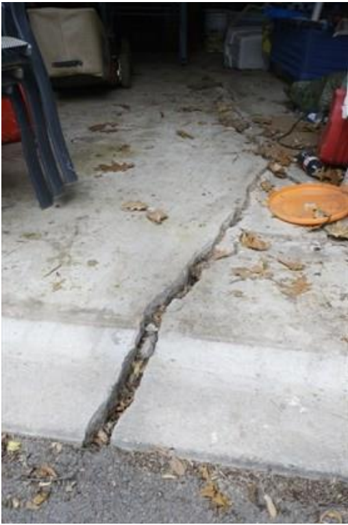
The garage floor of Donna Dobroski's home is being split by a crack.
