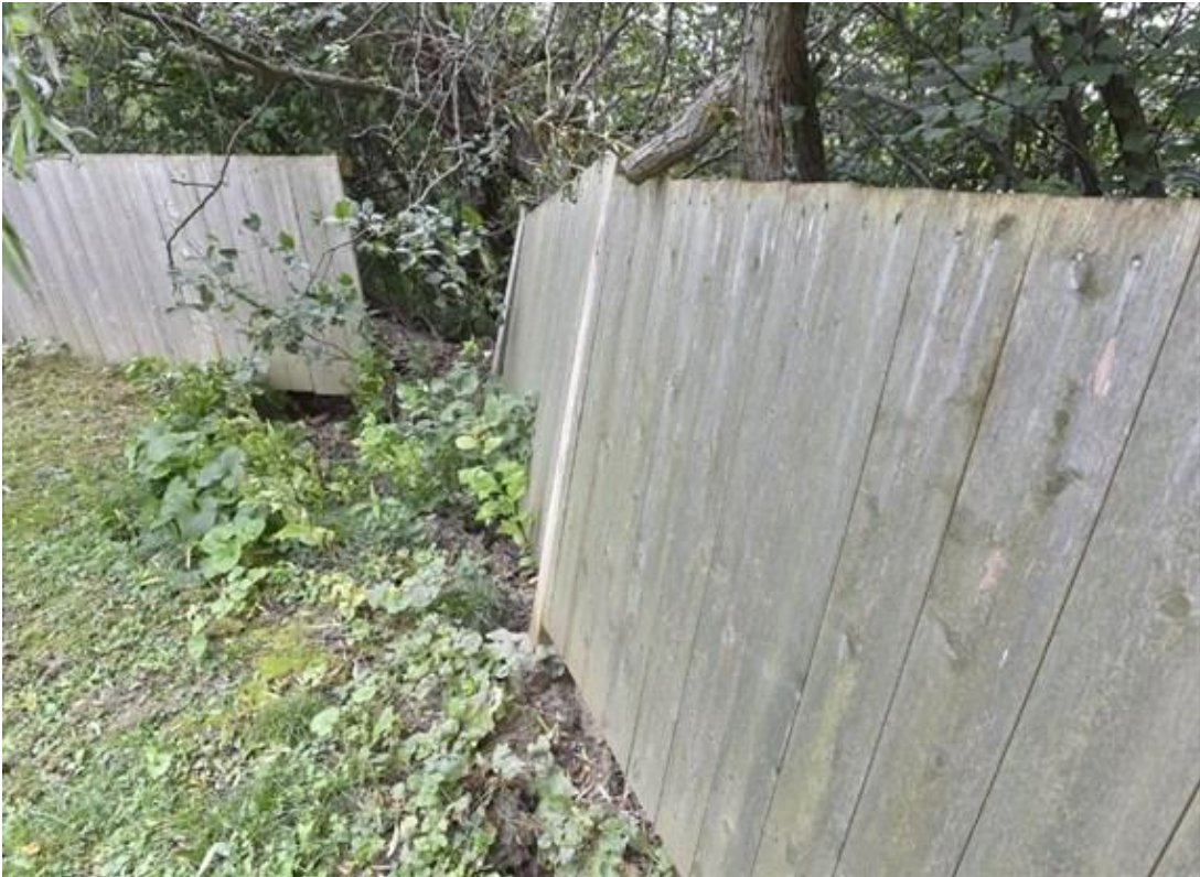
Donna Dobroski's fence is falling over due to erosion behind her house.
