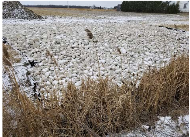
Almost complete grassed waterway & rock chute to reduce erosion
