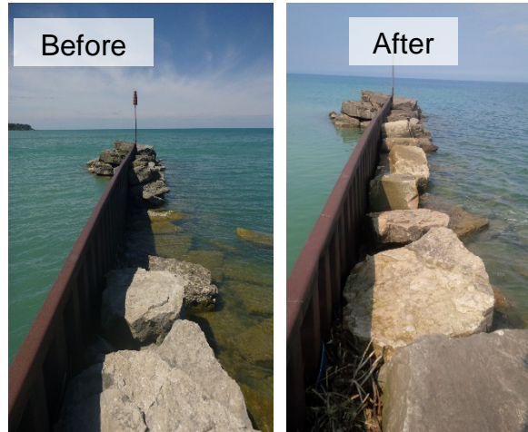
Armour stone seawall protection
