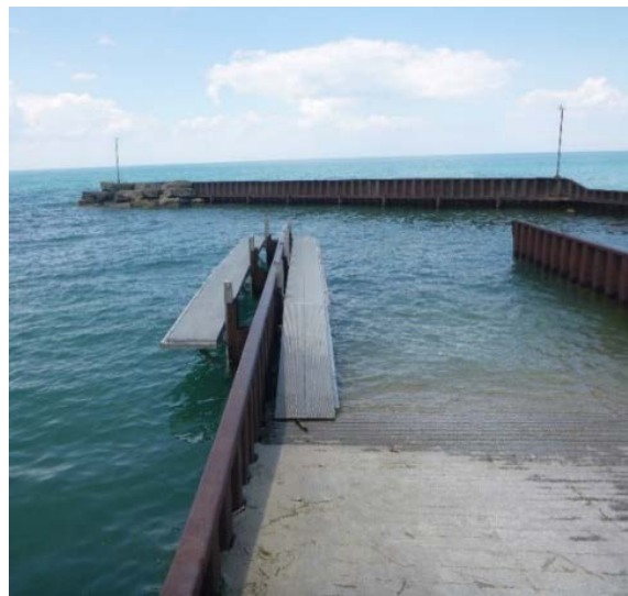
60' of new walkway along inside of boat ramp
