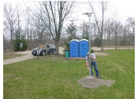
Solar light installation
