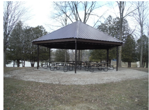
New steel roof on pavilion
