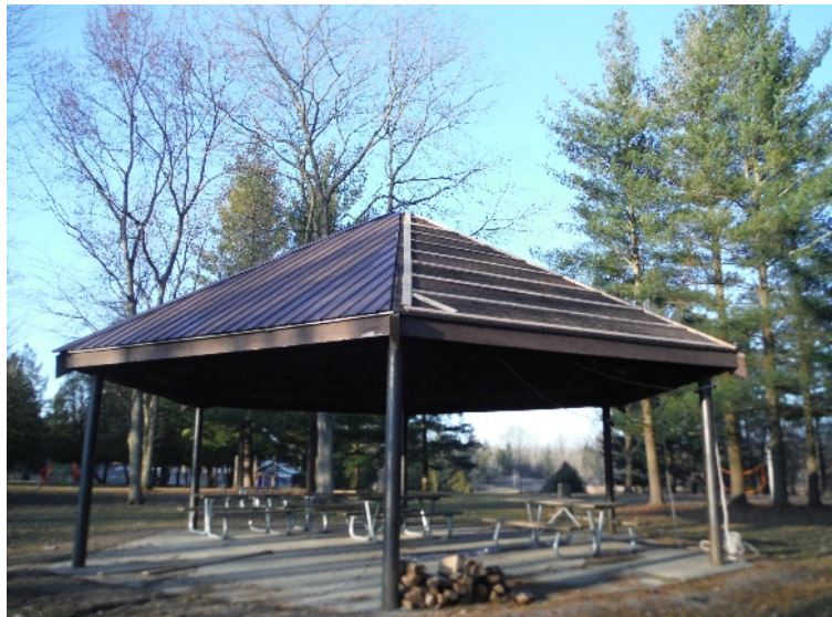
Steel roof being installed
