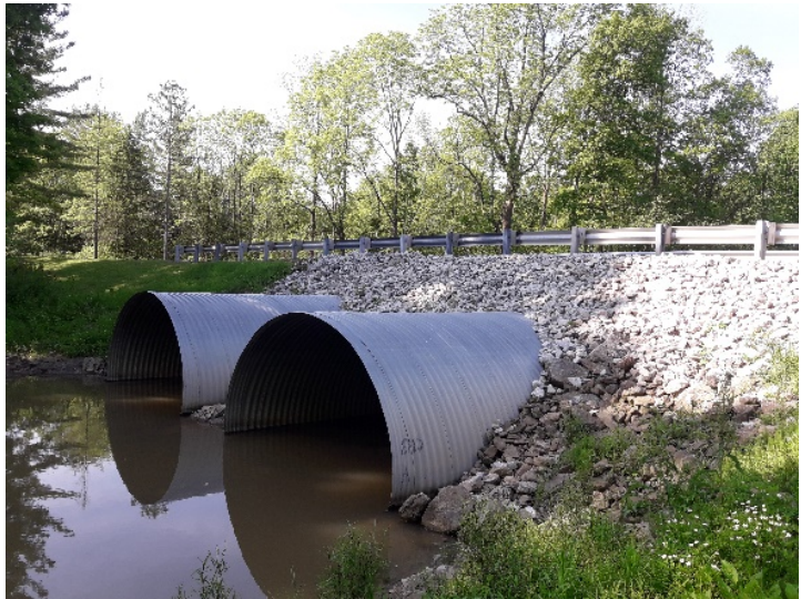
New riprap at road crossing
