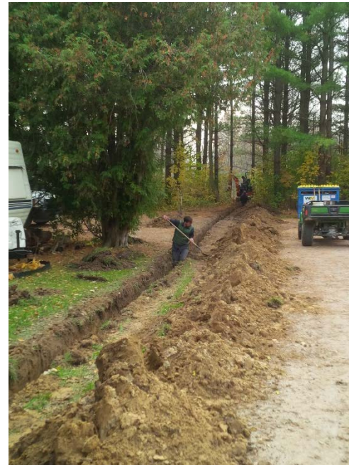
Warwick Drainage Installation
