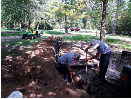
Drainage installation at Warwick CA
