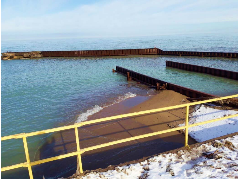
Sediment accumulation adjacent to the ramp.
