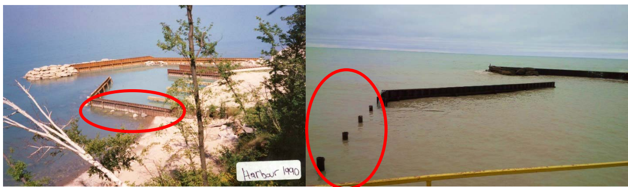
Highland Glen Ramp Protection 1990
