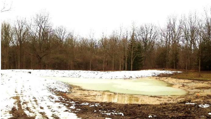
Wetland construction at Warwick CA
