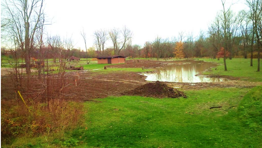
Wetland Construction at Bridgeview CA
