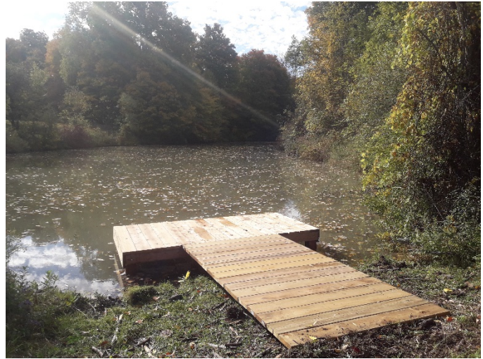
New dock at AWC
