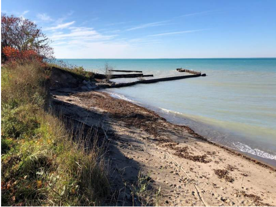
Photo 23- Looking East from Beach to Boat Launch
