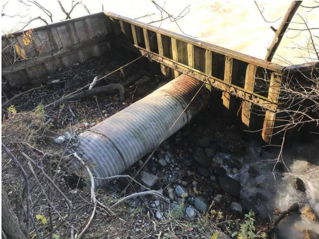
Photo 21- Exposed Corrugated Steel Pipe behind South Seawall Extension
