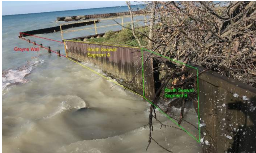
Figure 3. Groyne Wall (#1) and South Seawall (#2)
