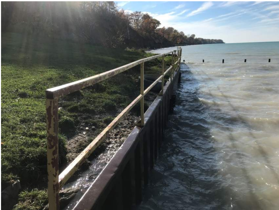
Figure 6. South Retaining Wall, Looking West
