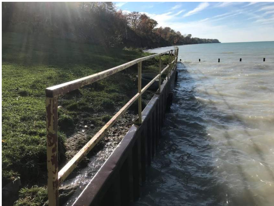
Photo 14- Looking West along South Retaining Wall
