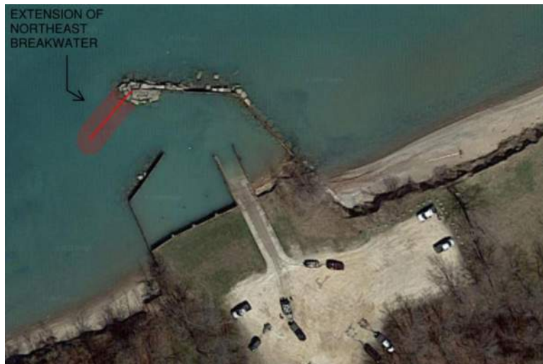
Figure 16 . Extension of Northeast Breakwater
