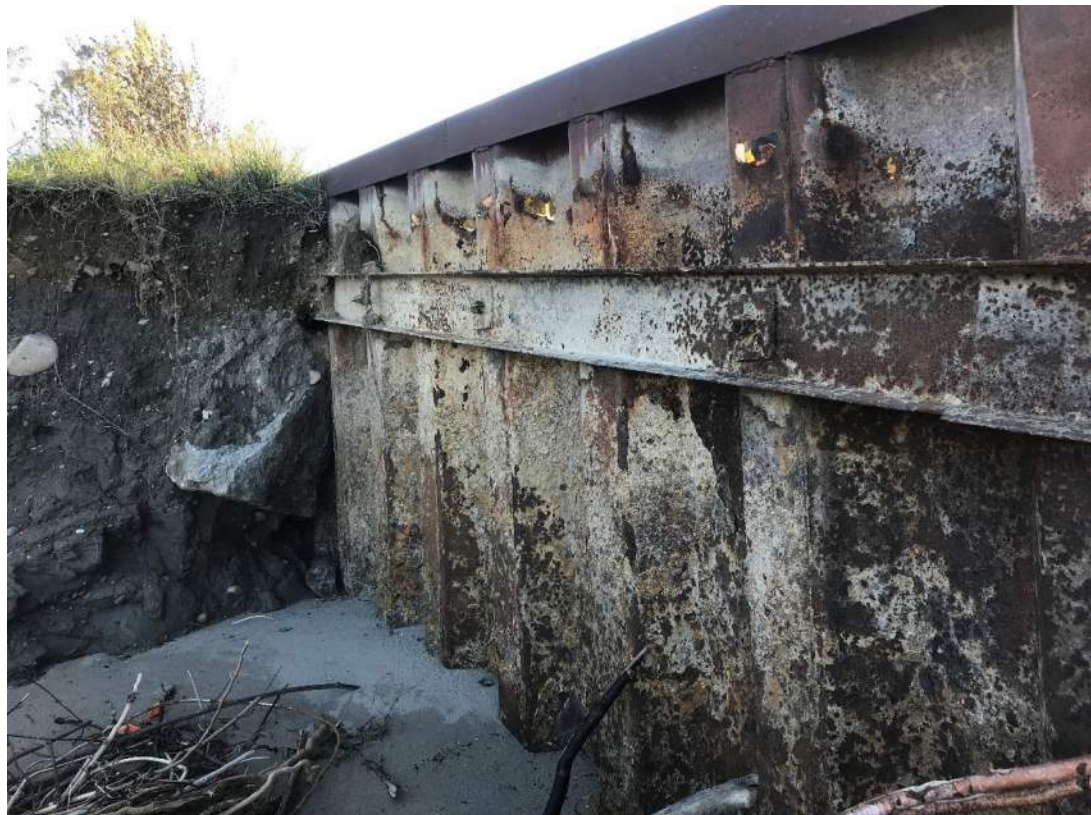
Photo 6- Outside of East Sheet Pile Wall, Boat Ramp
