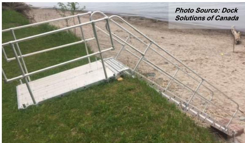
Figure 19. Removeable Stairway Example - Aluminum Stairway
