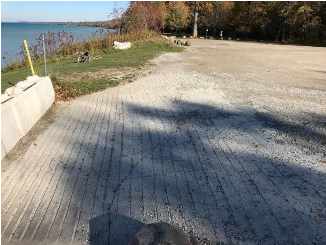
Photo 2- Top of Boat Ramp
