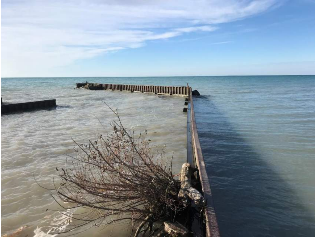
Photo 9- Northeast Curtain Wall
