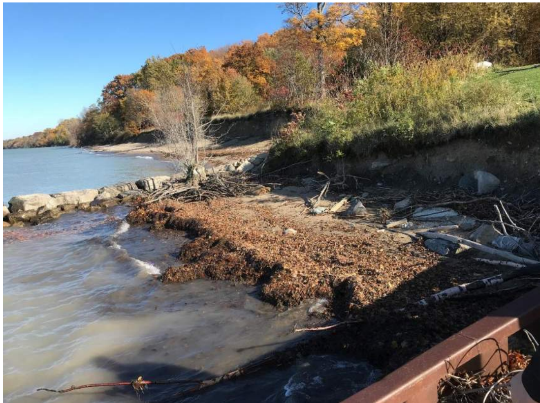
Photo 8- Erosion of Banks East of Boat Ramp
