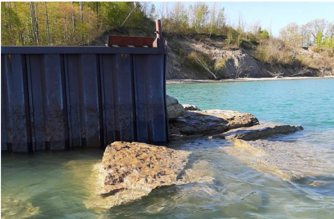
Photo 31- Lakeside of Northeast Breakwater looking East – Note deformation in wall near armour stone
