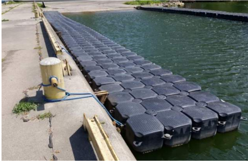
Figure 13. Modular Floating Platform
