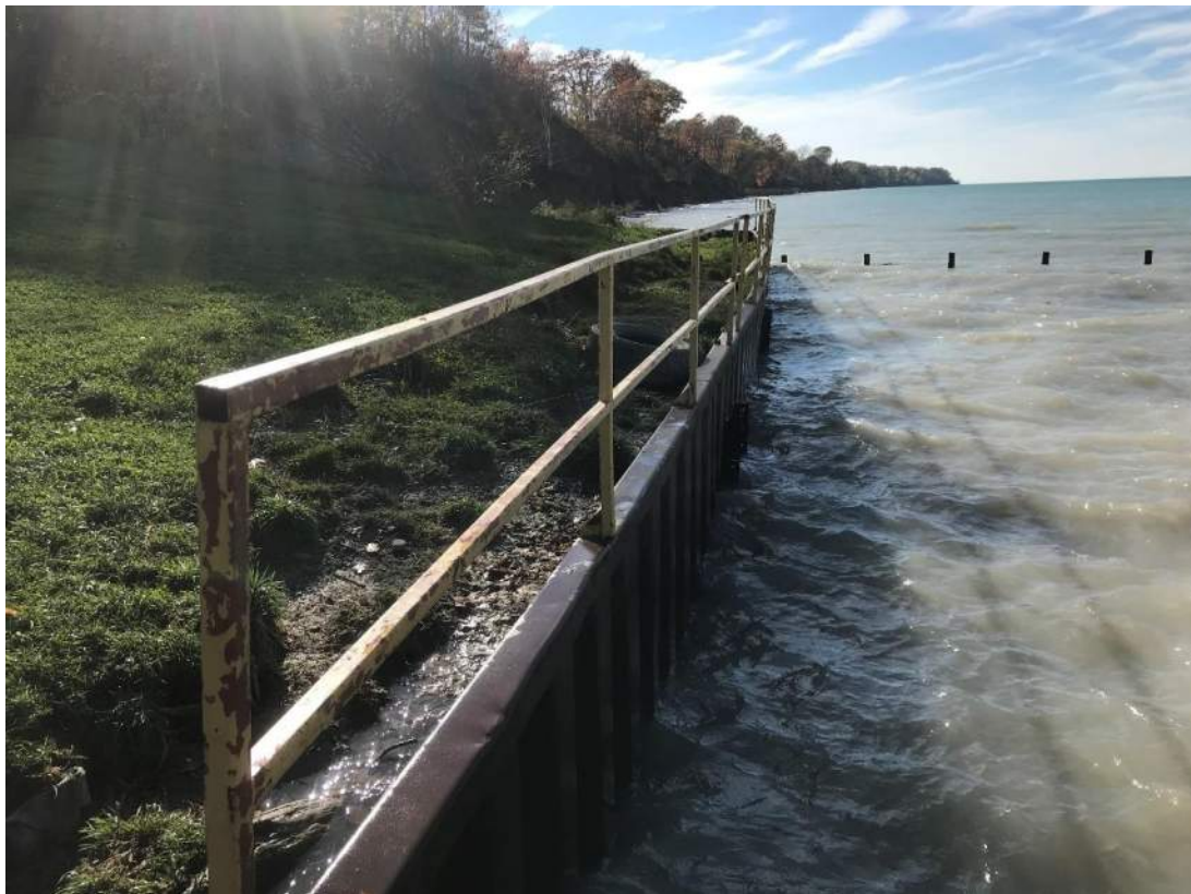
Photo 14- Looking West along South Retaining Wall
