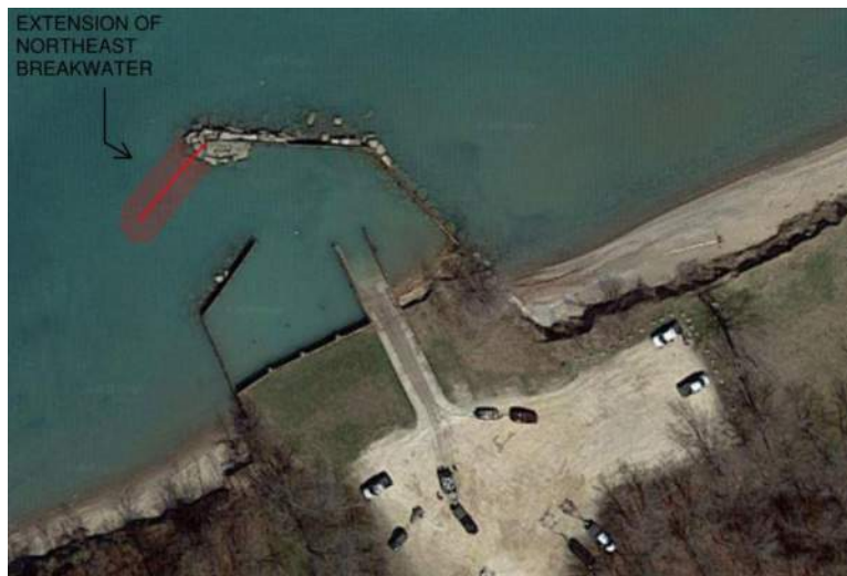
Figure 15 . Extension of Northeast Breakwater
