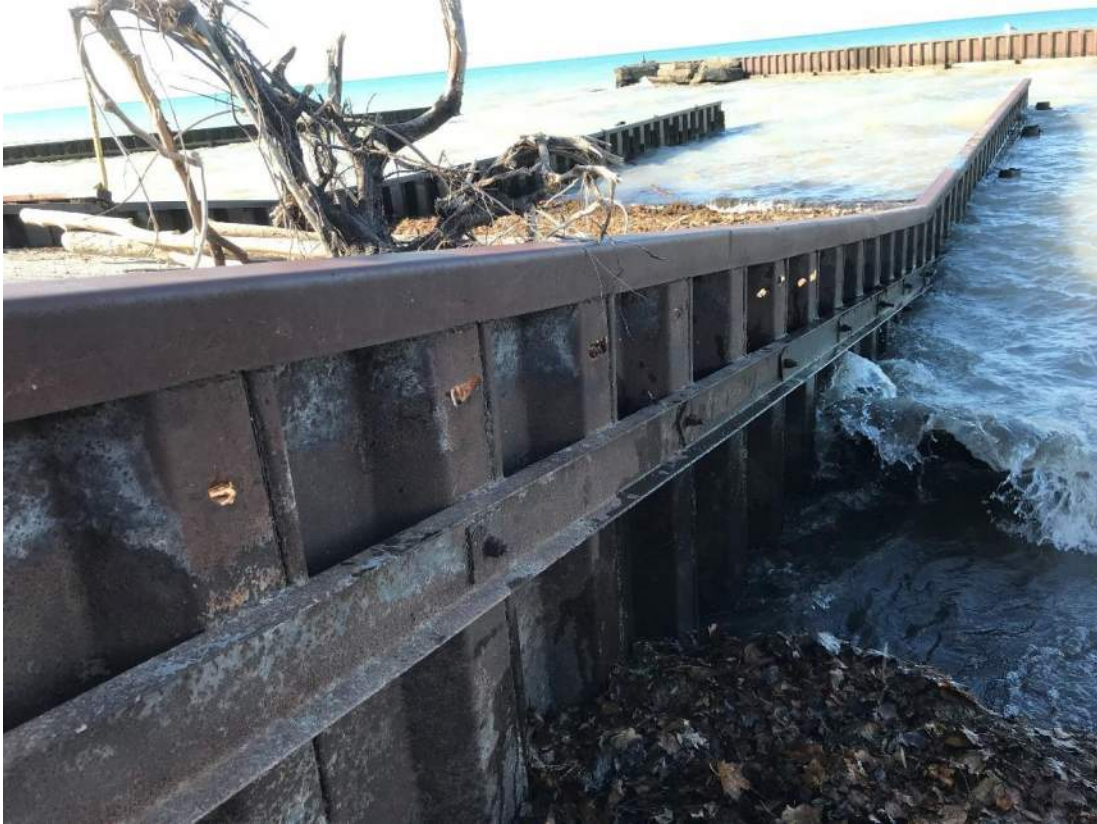
Photo 7- Outside of East Sheet Pile Wall, Boat Ramp
