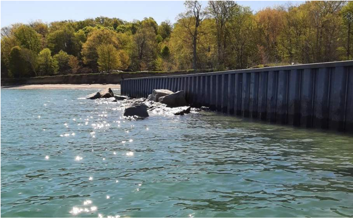
Photo 31- Lakeside of Northeast Breakwater looking East – Note deformation in wall near armour stone
