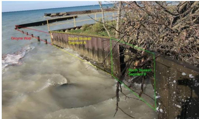
Figure 3. Groyne Wall (#1) and South Seawall (#2)
