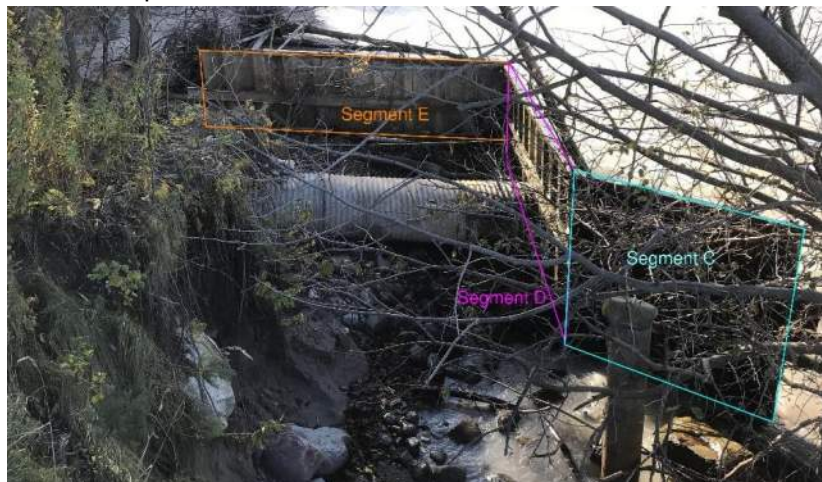
Figure 4. South Seawall Extension (#2) – Segments C, D and E
