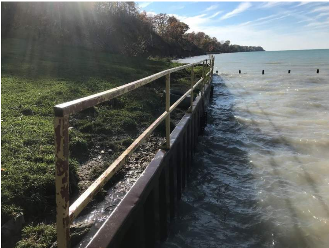
Figure 6. South Retaining Wall, Looking West
