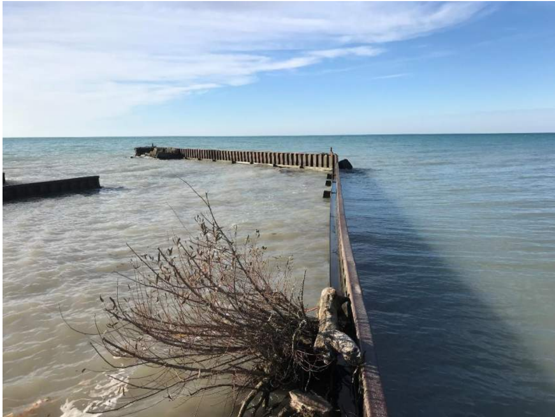
Photo 9- Northeast Curtain Wall
