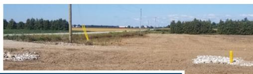
The completed WASCoB at the Gilroy property. The berm was designed to also serve as a continuation of the laneway. The yellow hickenbottom connects to an existing tile. The rock chute (far left in photo) slowly allows ponded water to enter the municipal drain.
