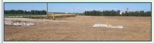
Recently completed and seeded low-level berm. This berm was designed to also serves as a continuation of the laneway. The hickenbottom connects to existing tile and the rock chute (at left of photo) slowly allows ponded water to enter municipal drain.
