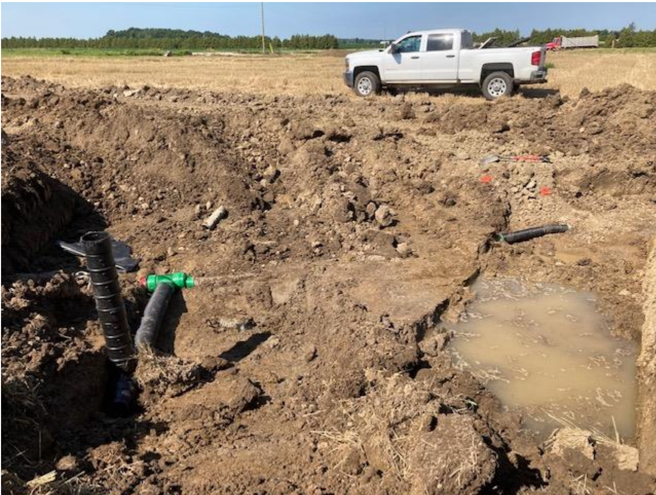
Attaching riser (hickenbottom) to existing tile
