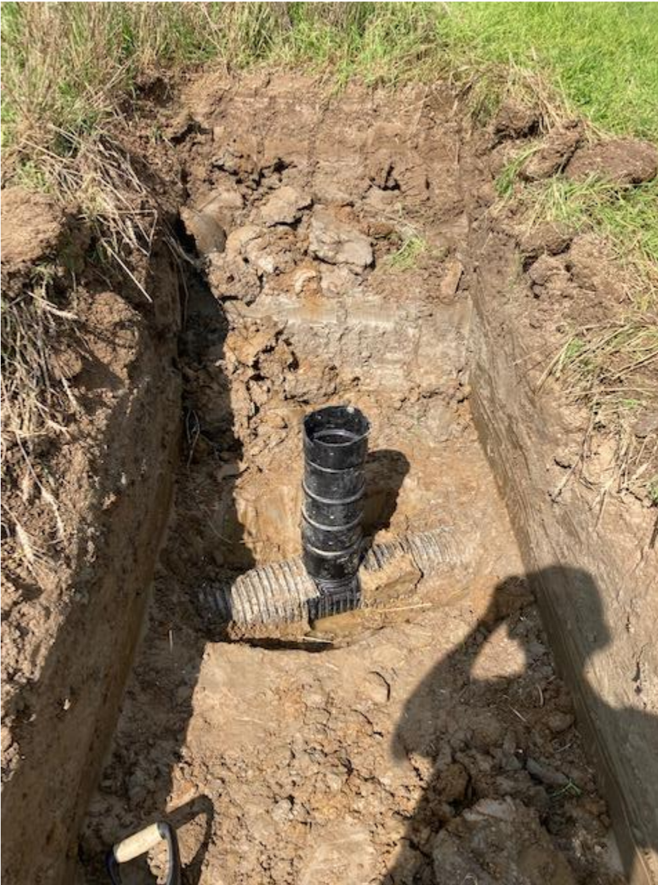
Photo of riser connection to tile
