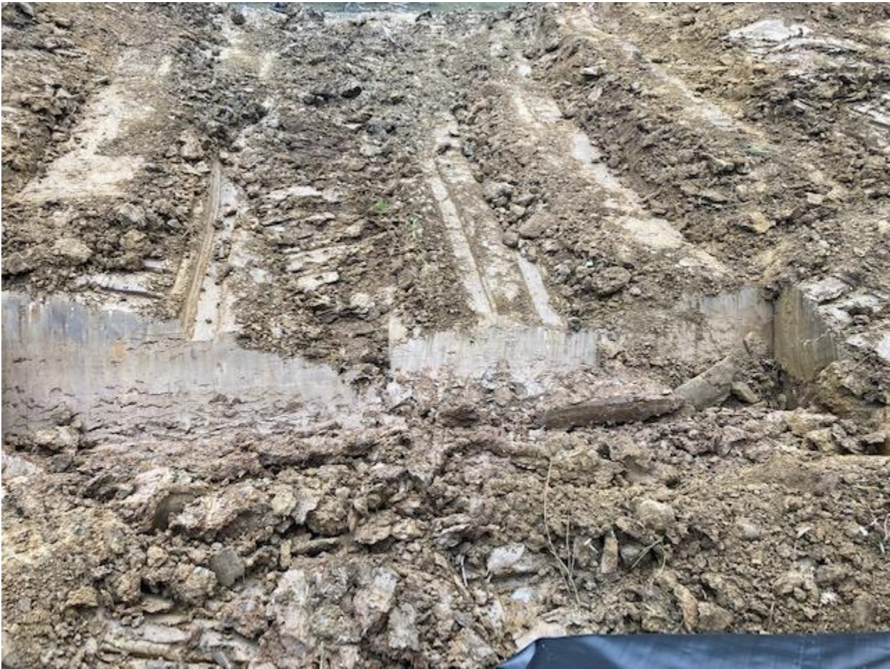
Notch at rock chute to hold riprap and geotextile fabric
