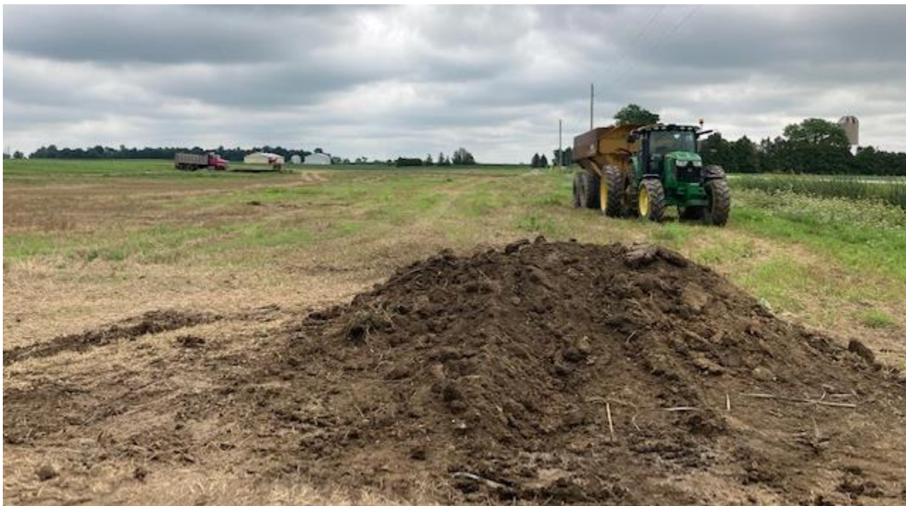
Photo of hauling subsoil from grassed waterway spoils to berms
