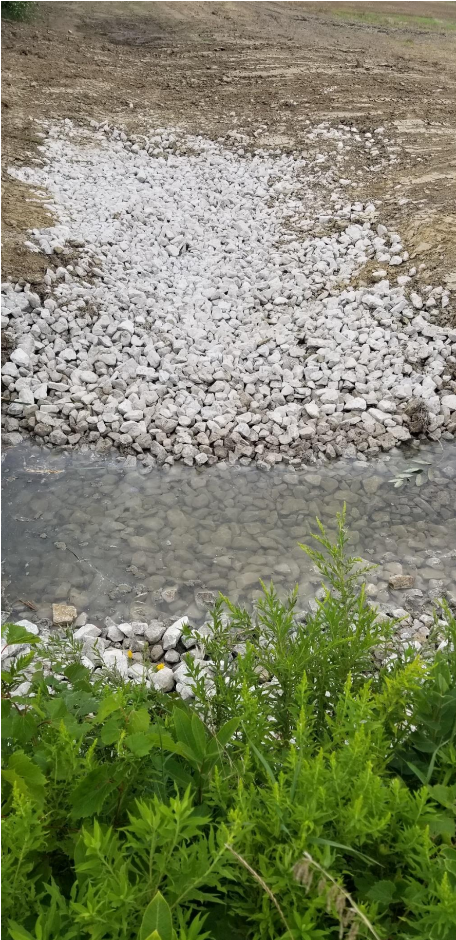
Photos of rock chute completed to specifications with apron into municipal drain
