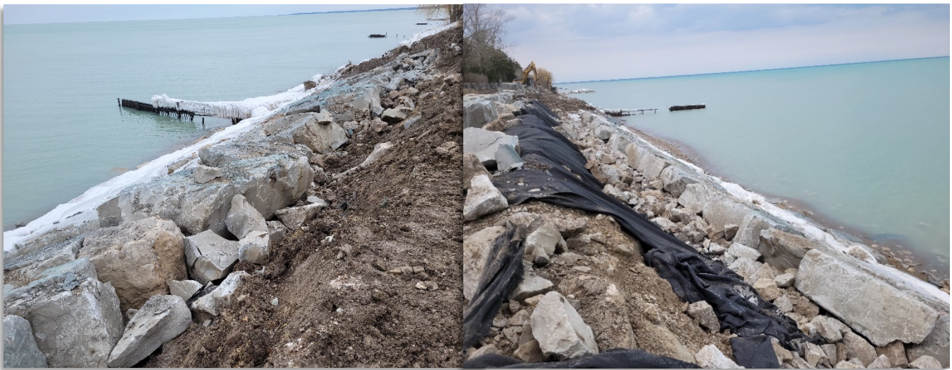
Pine St. to Penhuron Avenue – Shoreline construction progress
