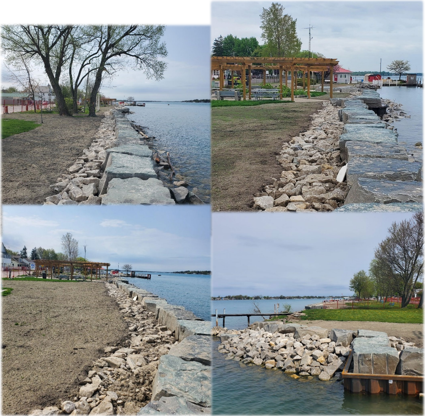
Port Lambton Park – Completed Shoreline project
