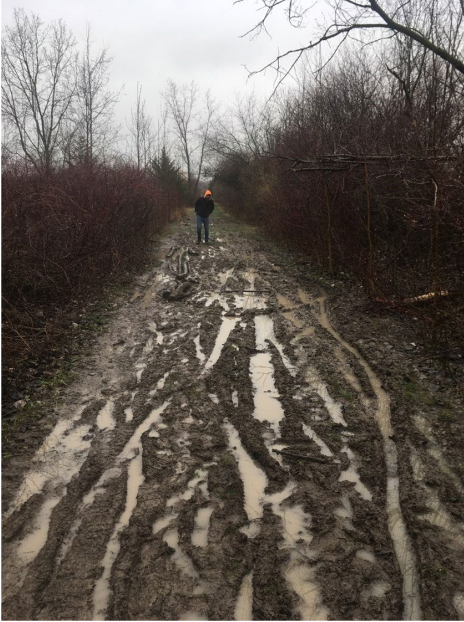
Above photo: trail condition this spring prior to closure
