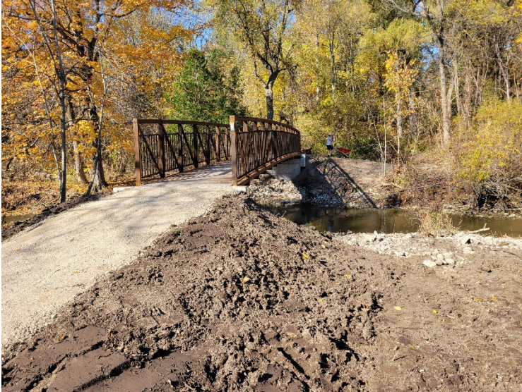
Left: New Coldstream Bridge
