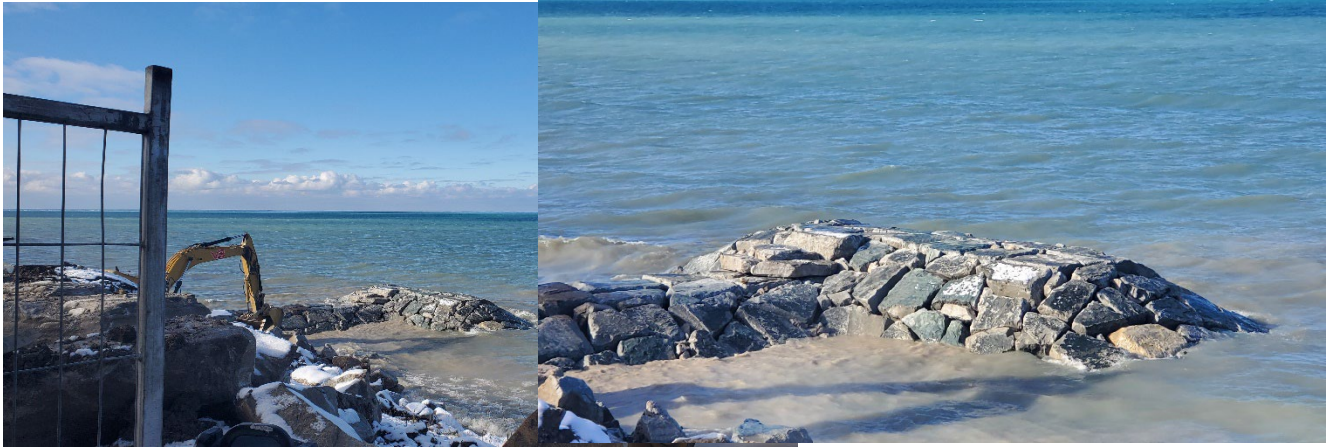
Penhuron avenue – Groyne installation
