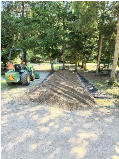
Gravel parking pad being installed at Warwick Conservation Area
