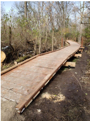
Above: Boardwalk replacement at Strathroy CA
