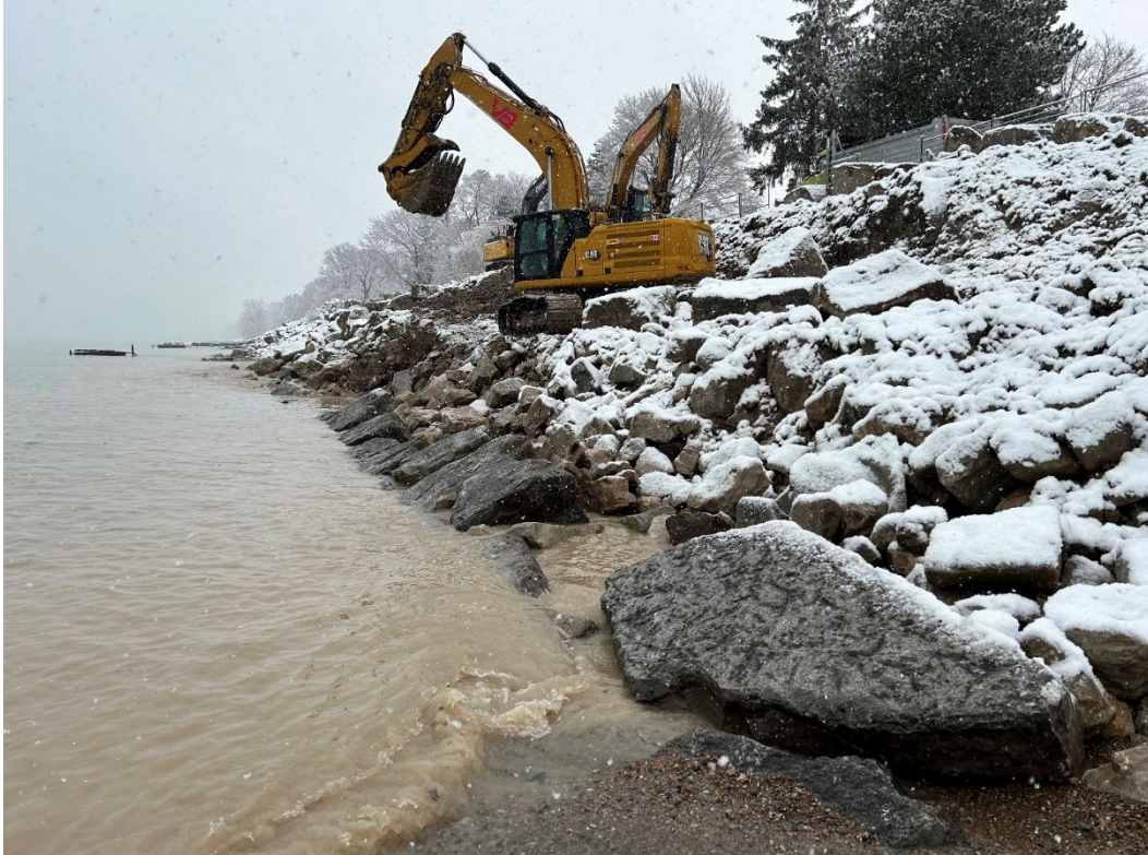
Construction Progress - Penhuron Drive to Kenwick Street Shoreline
