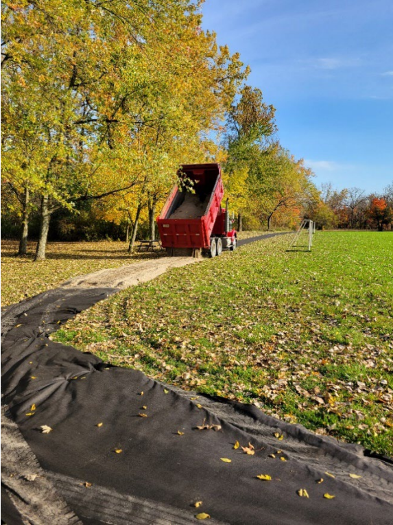
Above: Trail Installation
