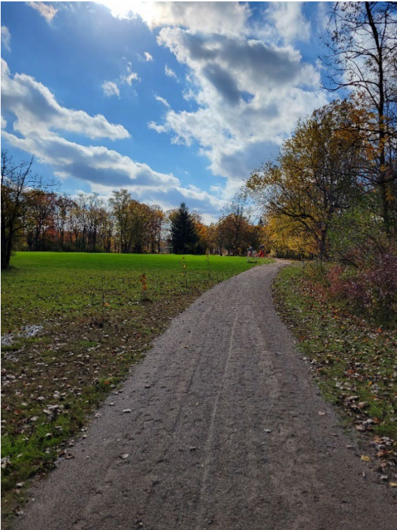
Above: Completed trail
