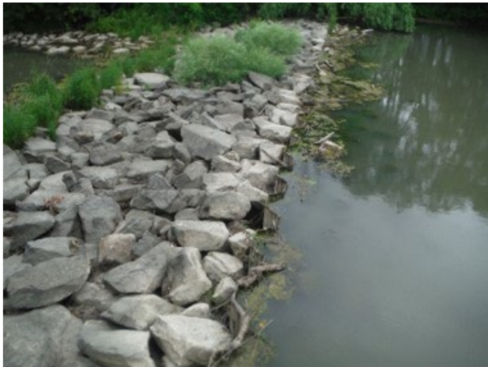
Photo 1: Head Street Dam vertical sheet piling and downstream armour stone.
