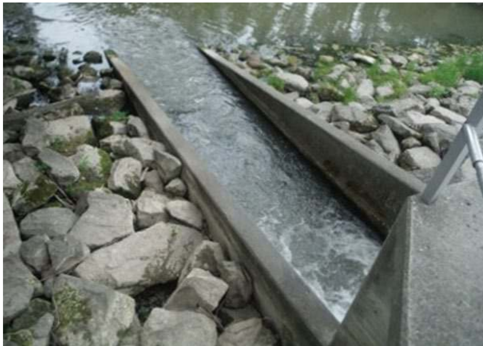
Photo 2: View of the Head Street Dam concrete spillway.
