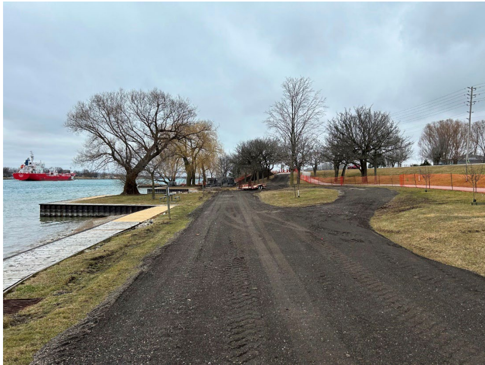
Seager Park – On site construction access preparation
