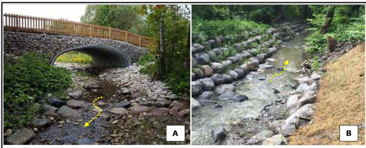
Figure 1: A) Typical vortex rock weir
