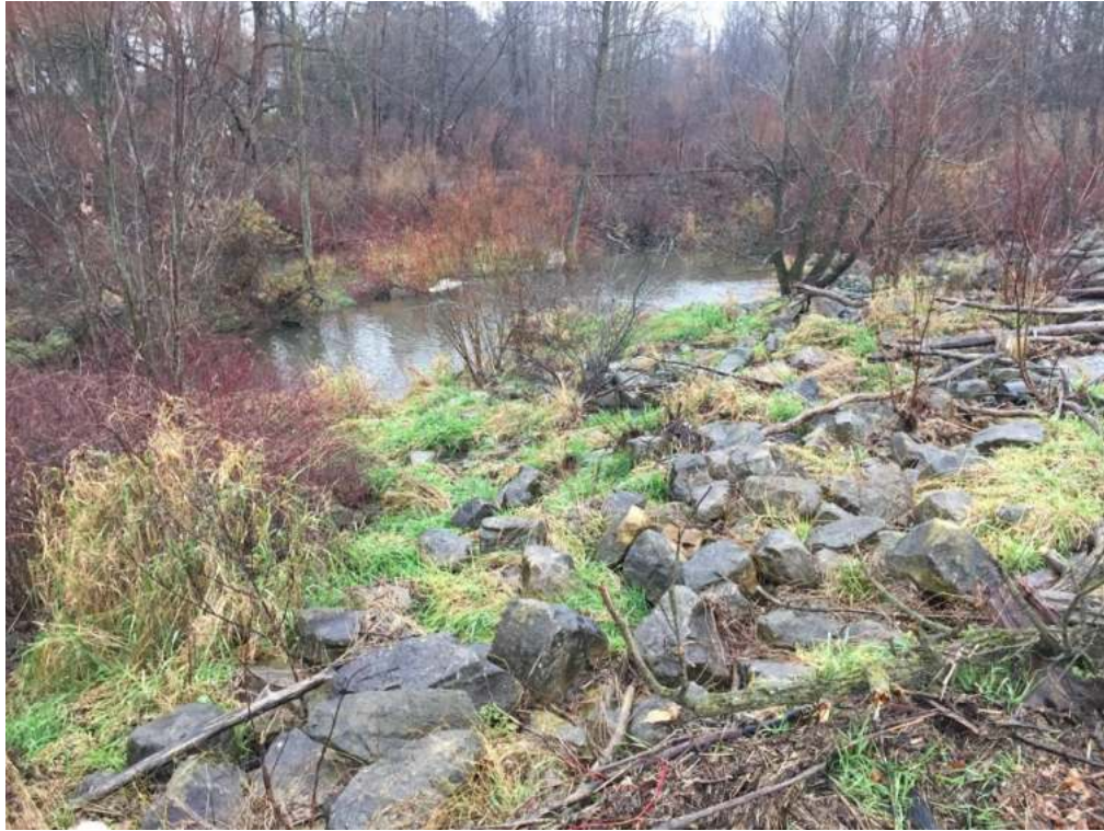
Photo 2: Large sloping armour stone placement on downstream side of sheet pile dam. Sydenham River downstream of dam visible in background.
