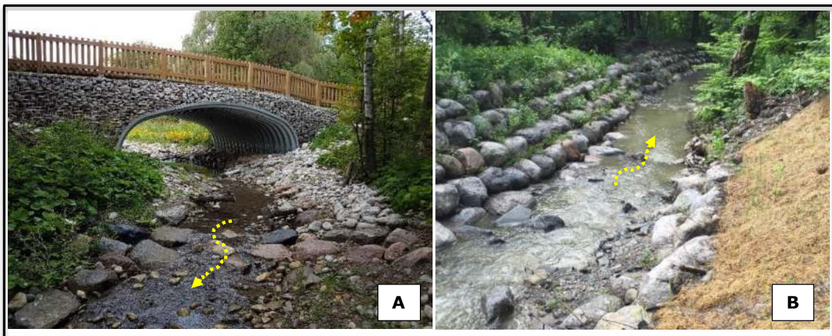
Figure 1: A) Typical vortex rock weir
