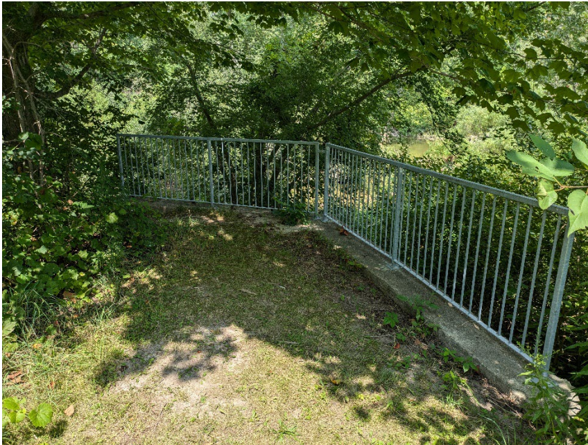
Above: new railings installed to mitigate fall risk at Coldstream CA
