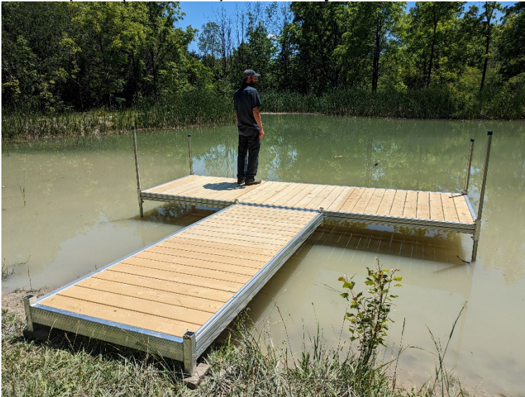
Above: new aluminum and cedar dock installed at Warwick CA
