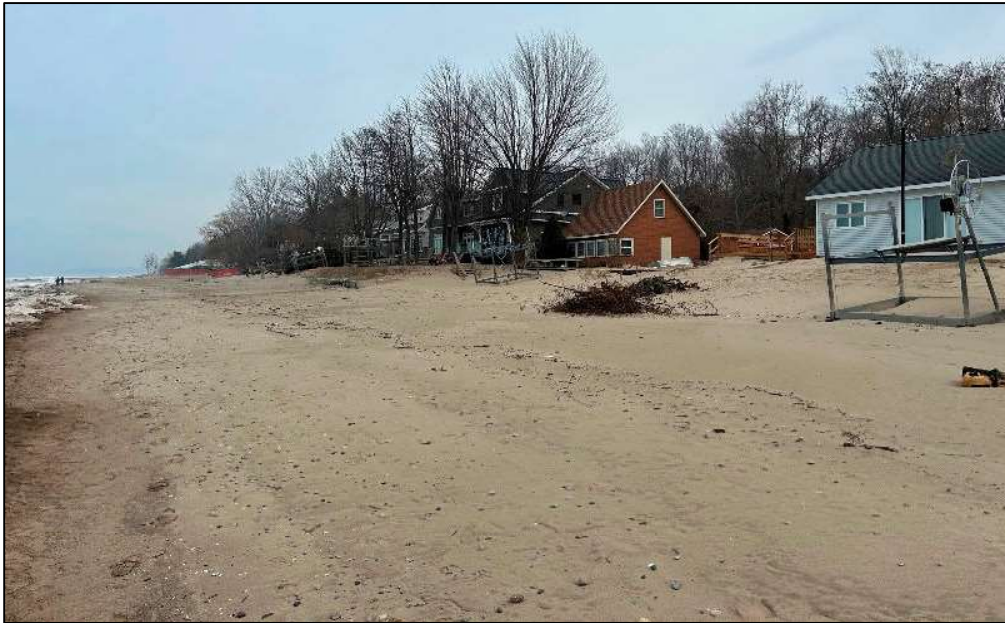
Photo 3 Northeasterly View of Adjacent Beach, February 2024
