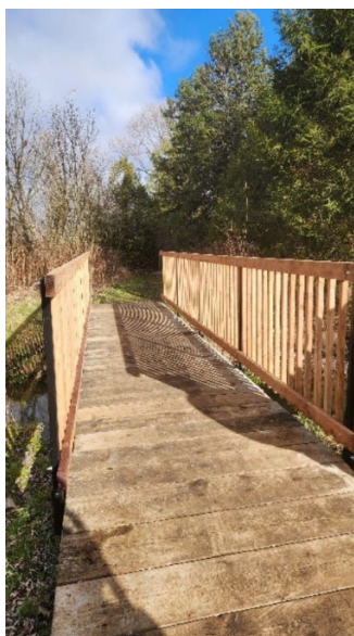
Above: Railings added to an existing bridge at Clark Wright CA
