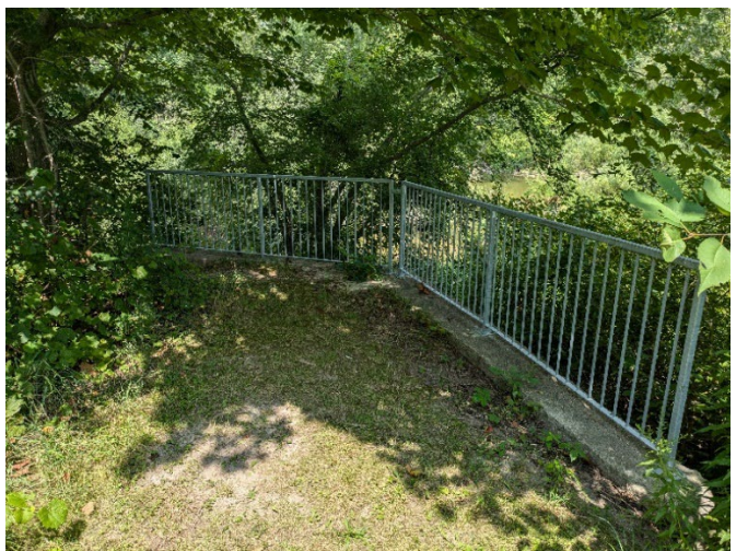
Above: Installation of safety railings
