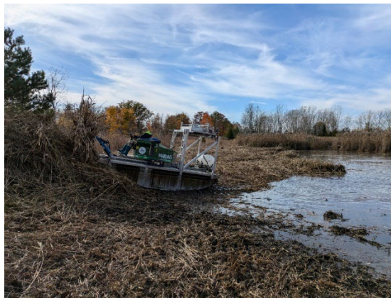
Above: Truxor unit piling cut phragmites
