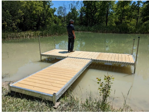
Above: New dock system installed
