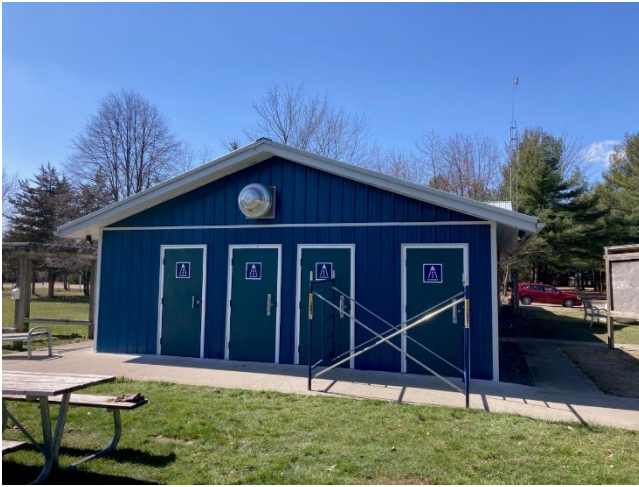
Above: Steel Siding installation
