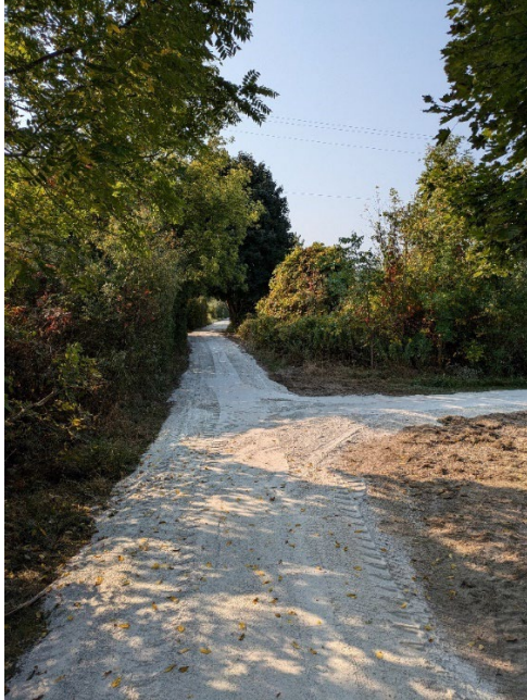
Above: Two photos of the stone dust trail installation at Wawanosh Wetlands CA
