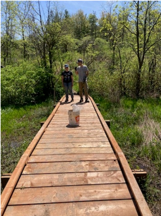
Above: Boardwalk installation
