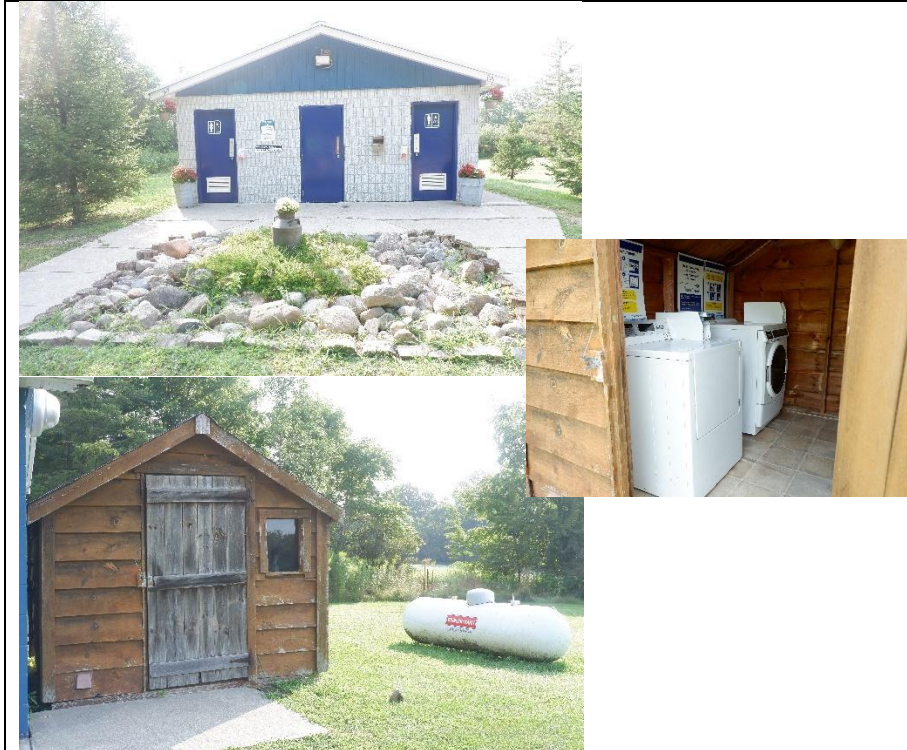
Main washroom building located south of seasonal camping, includes laundry facilities
